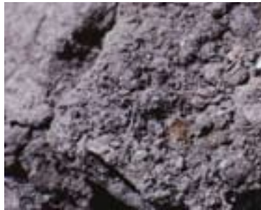
Why Test? Corrosive soils.
