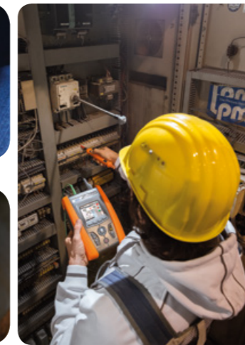
Start/stop measuring with remote lead PR400.
