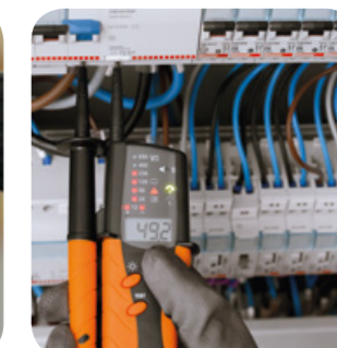
Measurement of phase sequence.
