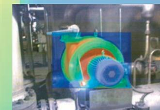
**Automatic Blend** A blend of the visual (visible light) and infrared image together to create a single image for optimal viewing. Easy menu options give you access to the different blending options from full thermal image to full visual image. Automatic blend provides enhanced detail to help locate problems precisely along with a visual frame of reference and helps to better focus the image.
