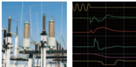
Application of each unit allows analysis of the correlation between voltage before and after the interruption of a generator, RPM fluctuation rate, governor servo motor operation conditions, and suppression machine switch timing.
