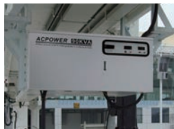
Airport Apron / Hangar
