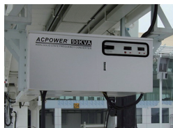
Airport Apron / Hangar
